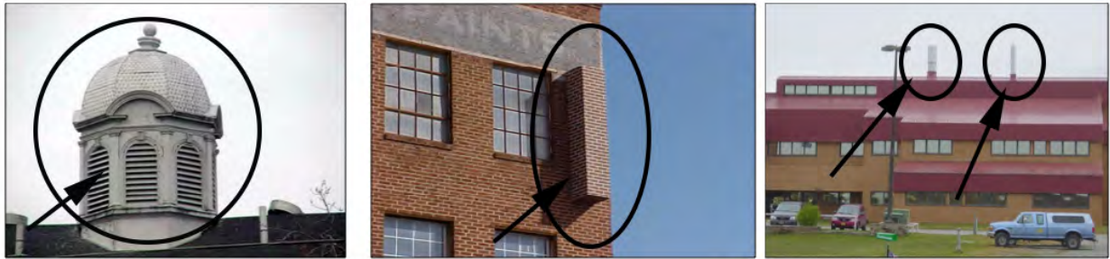
Figure 6: Examples of Antenna Concealment Techniques
