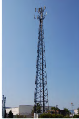
Self-Support Lattice Tower
