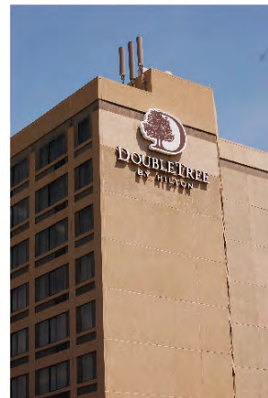
Figure 5: Examples of Non-Concealed Base Stations
