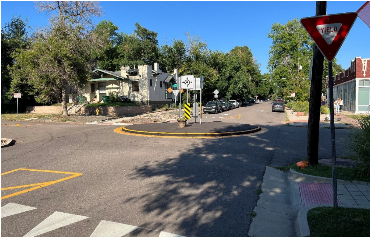
Mini roundabout on a Bicycle Boulevard.
